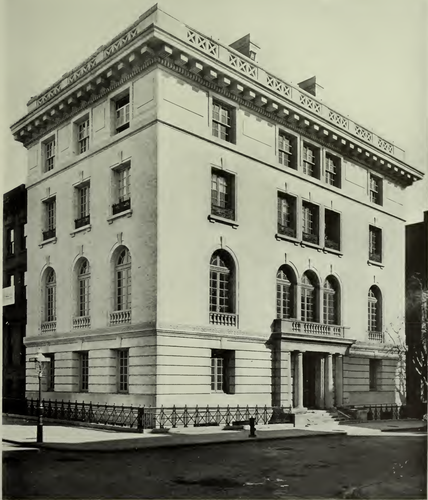
HOUSE, EIGHTY-FIFTH STREET AND PARK AVENUE, NEW YORK CITY. HUNT & HUNT, ARCHITECTS.
